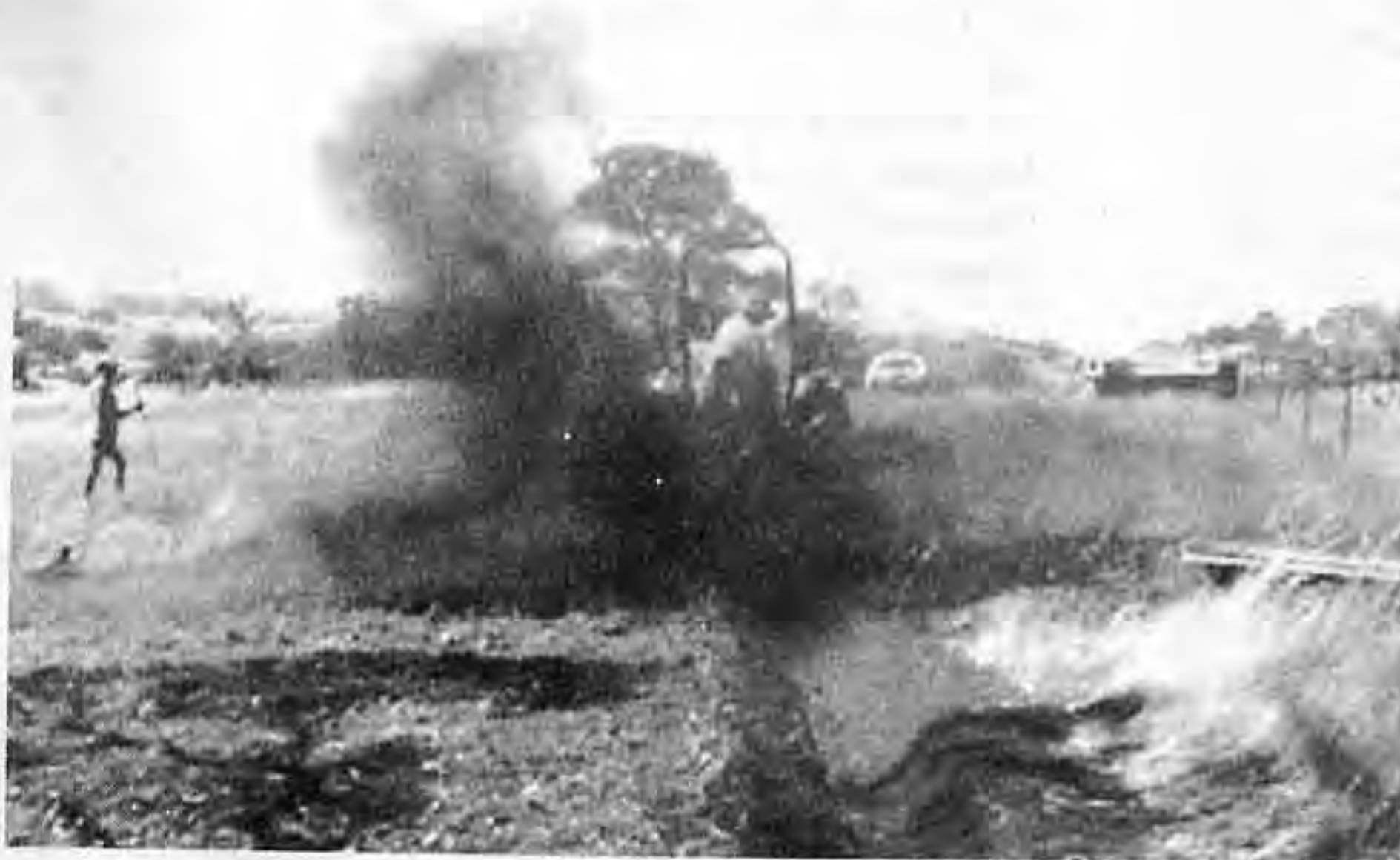
Making the dust fly: Cutting a drainage ditch with a channeller.
